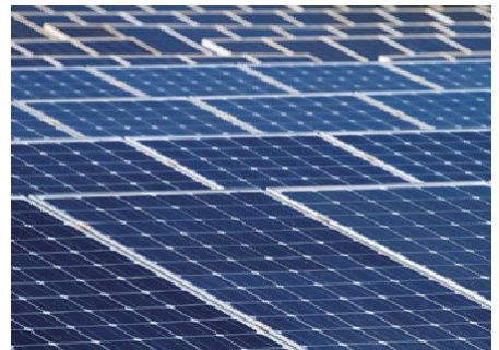
Solar Array Load Testing
