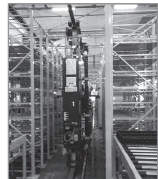
Automated Warehousing System
