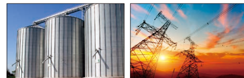
Hazardous Storage Tanks
